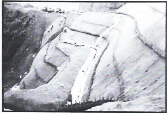
Use of Geo- mats for Slope Stabilization
