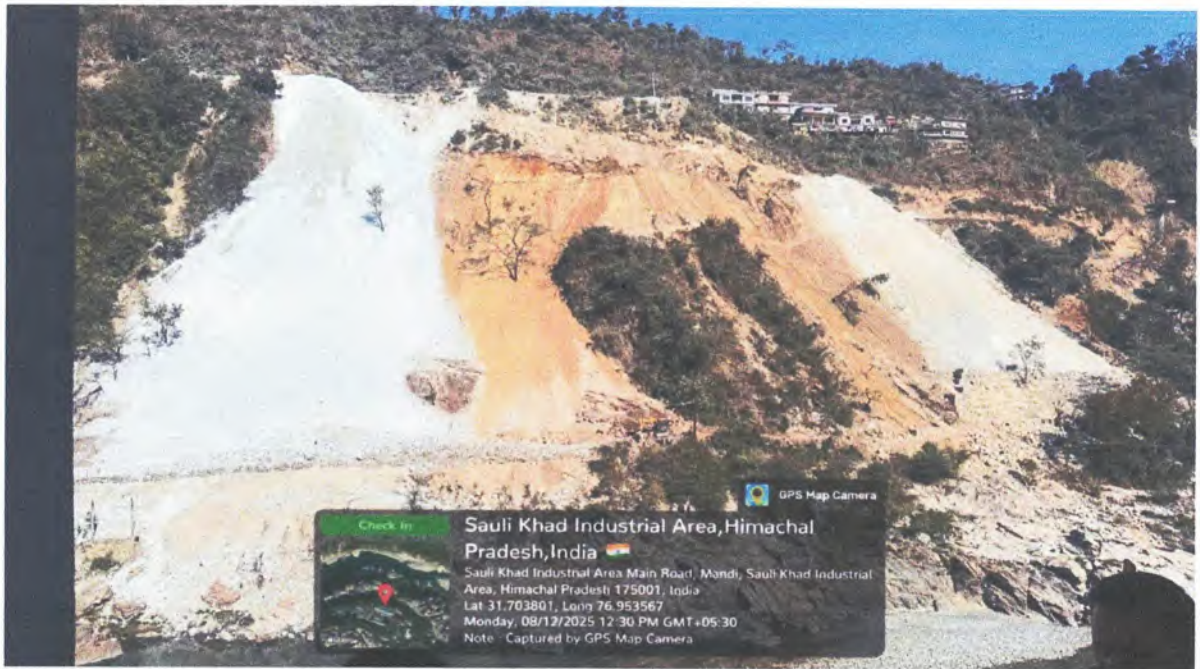
Photograph showing the Stretch of the Highway and the muck dumping Site
