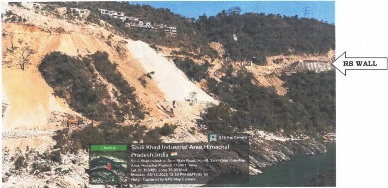
Photo P-4 Photograph showing the under-Construction RS Wall.
